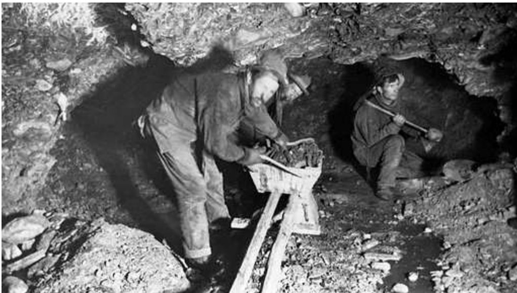
FIGURE 4: HAND SHAFTING AND DRIFTING IN BONANZA CREEK ON CLAIM 44 BELOW, 1901
